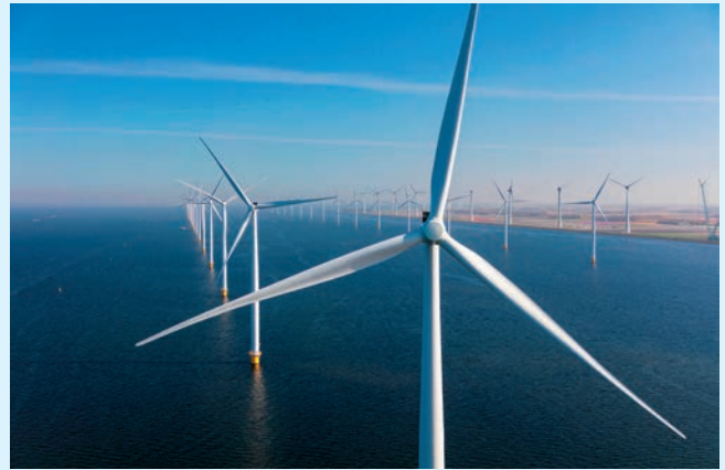
■ Figure A4.14 Wind turbines
