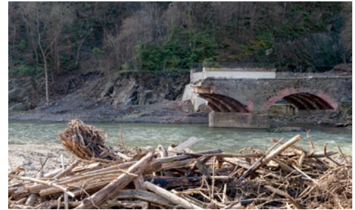
■ Figure B2.16 Flooding in Germany 2021
