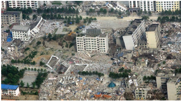
■ Figure C4.29 Resonance may be one reason why some buildings collapse in an earthquake
