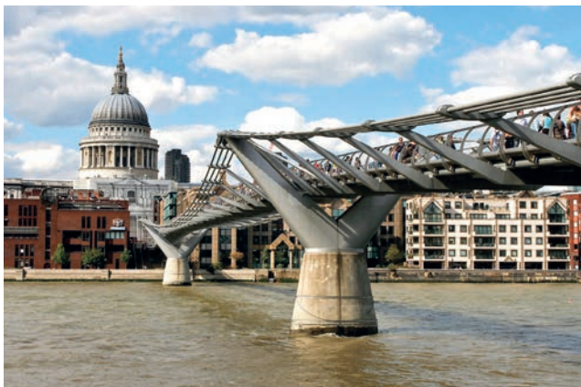
■ Figure C4.32 The Millennium Bridge in London was affected by resonance
