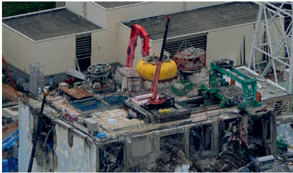
■ Figure E4.10 Fukushima nuclear reactor after explosions in the wake of the tsunami (2011)
