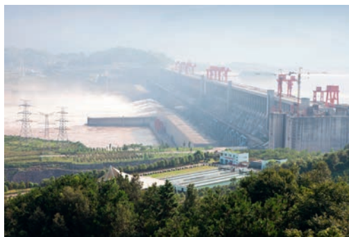
■ Figure A3.10 Water behind the Three Gorges Dam (China) stores enormous amounts of gravitational potential energy
