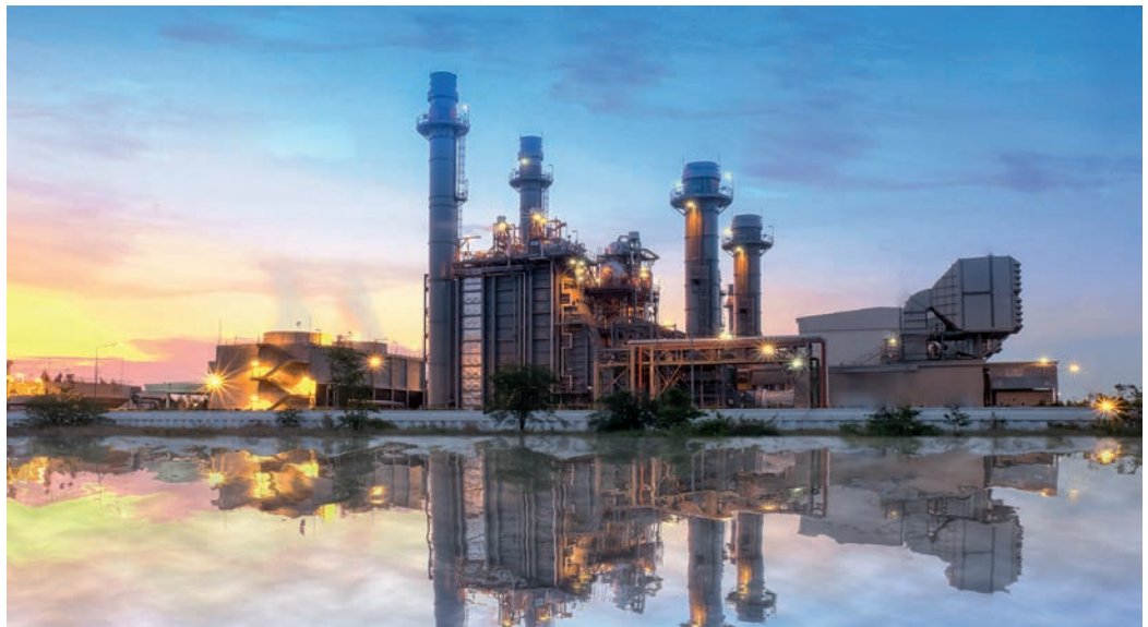
■ Figure A3.40 Power stations which use natural gas have the greatest overall efficiency ( \approx 60\% )
