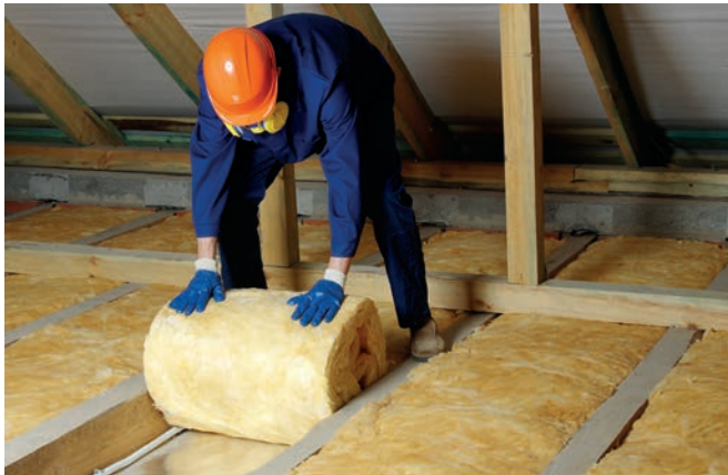
■ Figure B2.17 Improving insulation under the roof
