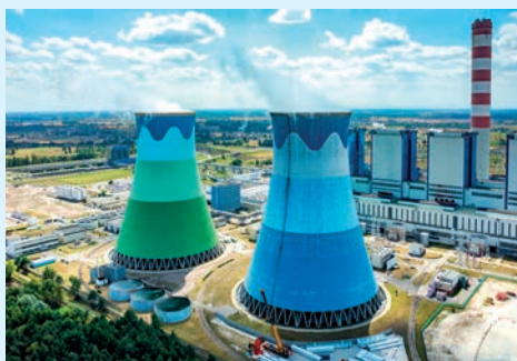
■ Figure B4.20 Cooling towers in Poland
